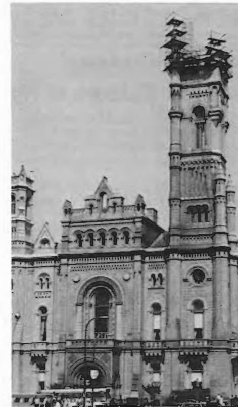
Masonic Temple, Philadelphia, is receiving a "face lifting." It will be completed by the September Quarterly Communication.
