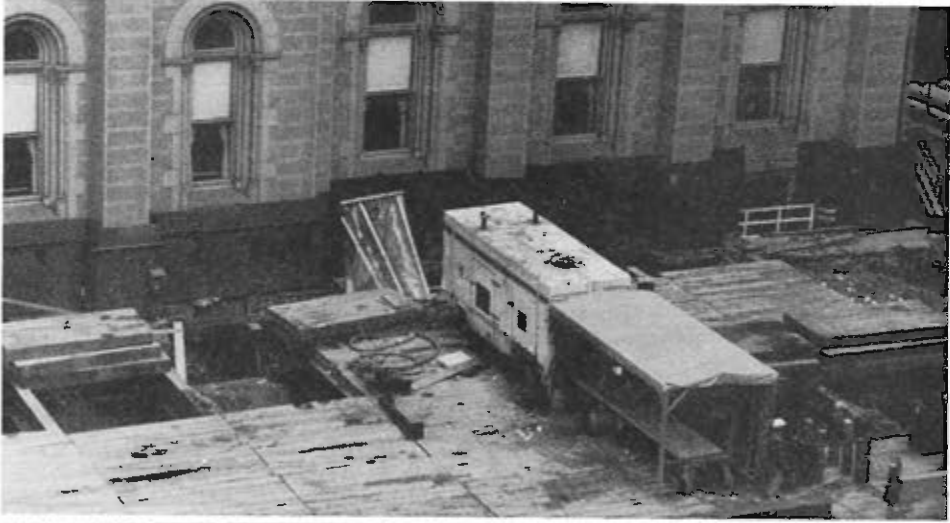
USING PHOTOGRAPHS TO TELL THE STORY —To better relate what is happening along the south wall of the Masonic Temple, Philadelphia, headquarters of our Grand Lodge, the photograph above shows the extent of activity and excavation on the Center City Commuter Tunnel. The photograph below is a close-up showing that the soil has been removed right up to the original foundation of the Temple which was laid in 1868. The accompanying article covers more detail on this unfortunate experience.
