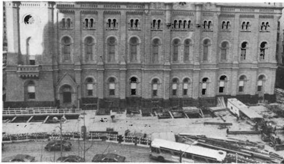
USING PHOTOGRAPHS TO TELL THE STORY —To better relate what is happening along the south wall of the Masonic Temple, Philadelphia, headquarters of our Grand Lodge, the photograph above shows the extent of activity and excavation on the Center City Commuter Tunnel. The photograph below is a close-up showing that the soil has been removed right up to the original foundation of the Temple which was laid in 1868. The accompanying article covers more detail on this unfortunate experience.
