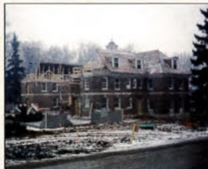
The roof on the back of the Brown building is removed in preparation for the addition to the building.
